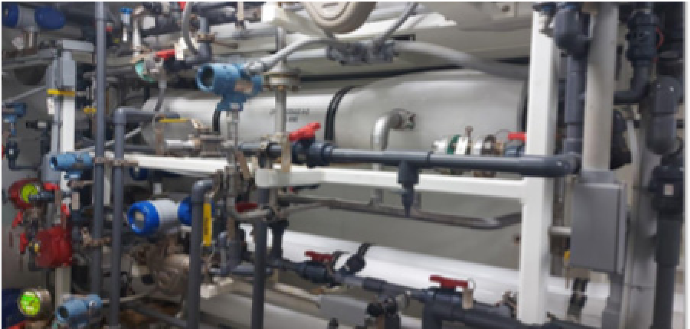
Figure 3: The above selected photos shows the existing CFRO system, within the pilot plant operated by SAWACO.
